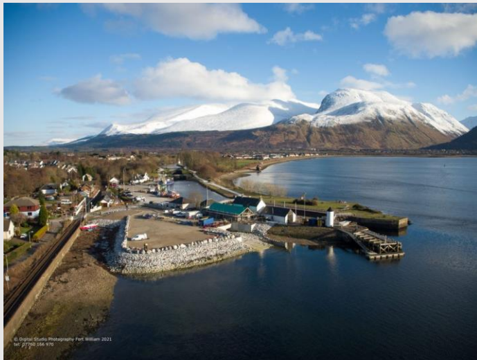
Corpach Marina Project
